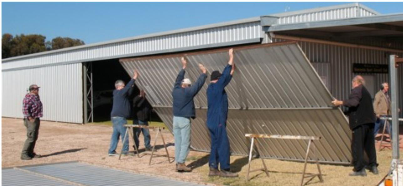
An excellent turn-up to a working bee held on Sunday 17th August made short work of modifying two troublesome doors on the Club's No 1 Hangar. Reducing the height of the door panels slightly and fitting new carriage wheels did the trick. That's Peter Guest in full protective head-gear on the left directing proceedings. Below: "Cut it about there I reckon". The experts at work. Many thanks to all who turned out to help.
